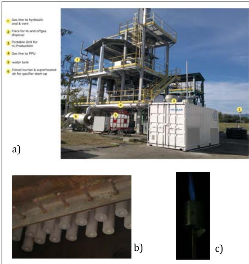
Fig3 UNIfHY integrated plant at the ENEA-Trisaia Research Centre: a) facility coupled to the portable purification unit (PPU) for gas conditioning and H<sub>2</sub> separation; b) view detail of the in-situ HT filtration system; c) gas disposal flare, fed by the produced H<sub>2</sub> and the off-gas streams from the PPU
