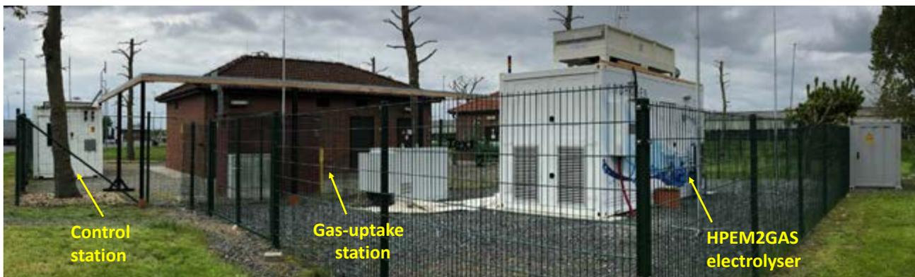
Fig.2 HPEM2GAS power-to-gas plant in Emden, Germany. On the right, the high performance 200 kW electrolyser from ITM Power based on Solvay Aquivion® membrane and CNR-ITAE electrocatalysts (HPEM2GAS project).
