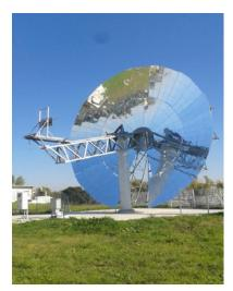
Fig. 3 Parabolic dish receiver at the ENEA Casaccia Research Centre
