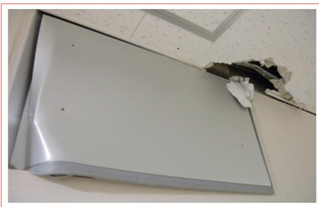
**PHOTO 3** Damage to cover panel
