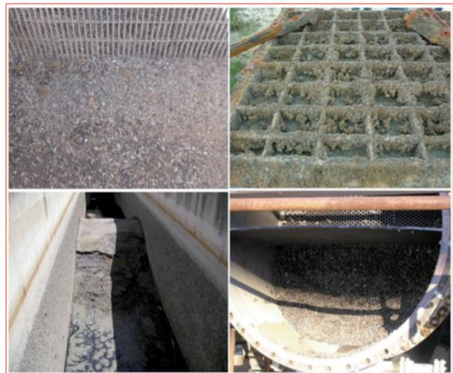
**FIGURE 2** Biofouling colonization residual inside cooling water system [1]
