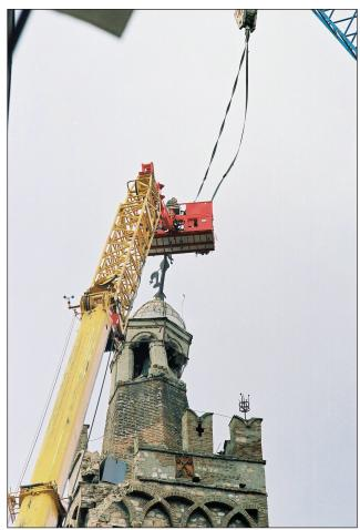
FIGURE 3 Securing the Torrino in Foligno, following the 1997 earthquake
