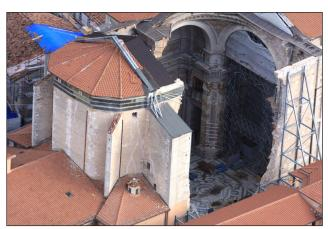
FIGURE 10 Securing the Duomo in L'Aquila, following the 2009 earthquake
