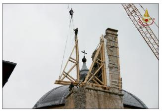
FIGURE 5 Securing the bell gable of the Basilica di S. Bernardino in L'Aquila, following the 2009 earthquake
