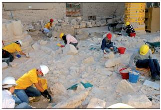
FIGURE 6 Restoration and screening of the ruins in the Church of S. Maria di Collemaggio in L'Aquila, following the 2009 earthquake
