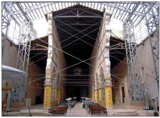
FIGURE 7 Securing and roofing the transept in the Church of S. Maria di Collemaggio in L'Aquila, following the 2009 earthquake
