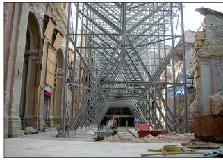
FIGURE 9 Securing and roofing the Church of S. Maria di Paganica in L'Aquila, following the 2009 earthquake Source: Author's personal archive
