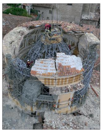
FIGURE 8 Securing the dome of the Church of S. Maria del Suffragio in L'Aquila, following the 2009 earthquake Source: Author's personal archive
