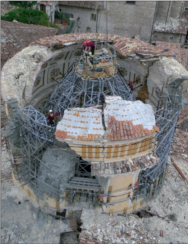
**FIGURE 8** Securing the dome of the Church of S. Maria del Suffragio in L'Aquila, following the 2009 earthquake
