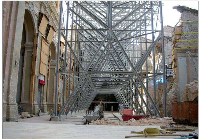
**FIGURE 9** Securing and roofing the Church of S. Maria di Paganica in L'Aquila, following the 2009 earthquake
