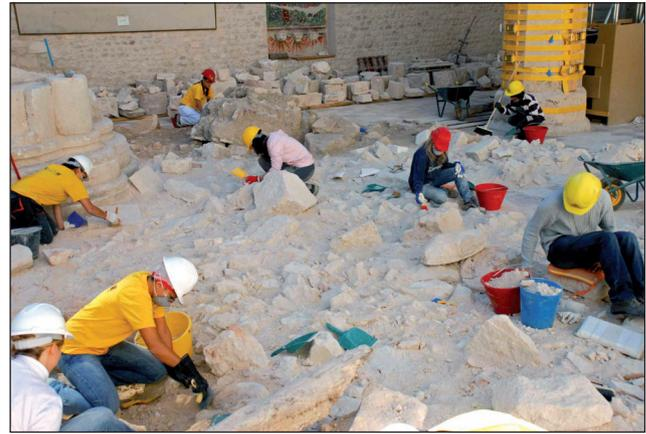
**FIGURE 6** Restoration and screening of the ruins in the Church of S. Maria di Collemaggio in L'Aquila, following the 2009 earthquake
