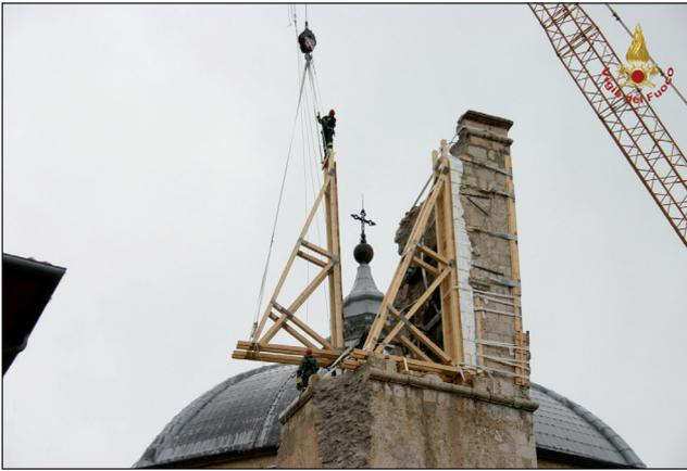
**FIGURE 5** Securing the bell gable of the Basilica di S. Bernardino in L'Aquila, following the 2009 earthquake
