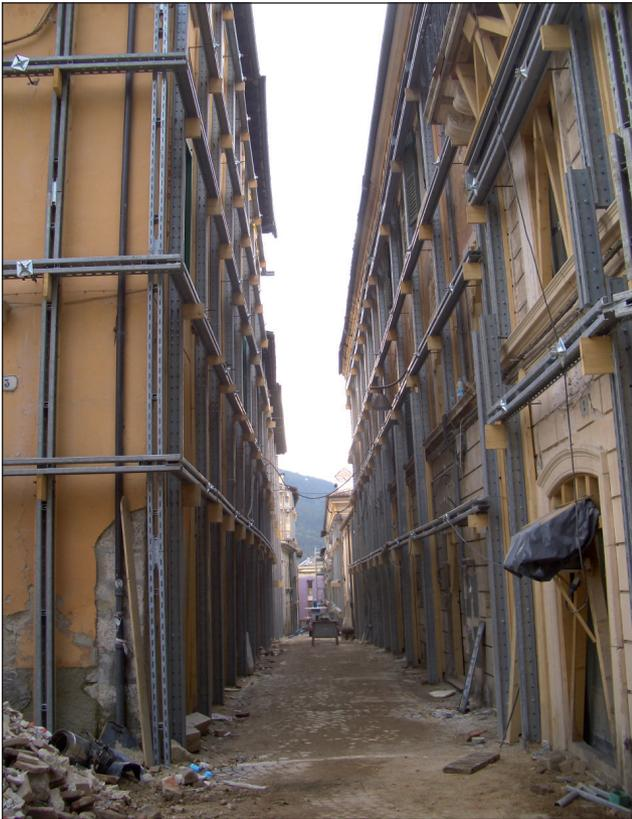
**FIGURE 11** Securing historical palaces in the historical centre of L'Aquila, following the 2009 earthquake
