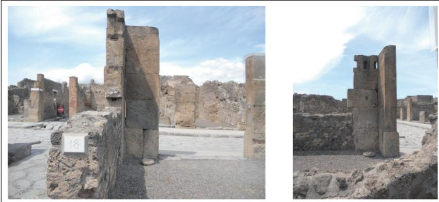
**FIGURE 8** Stacked blocks of tuff for the case study
