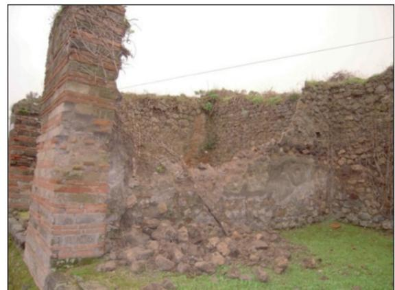
**FIGURE 5** Walls showing different structural behaviors and resultant damage
