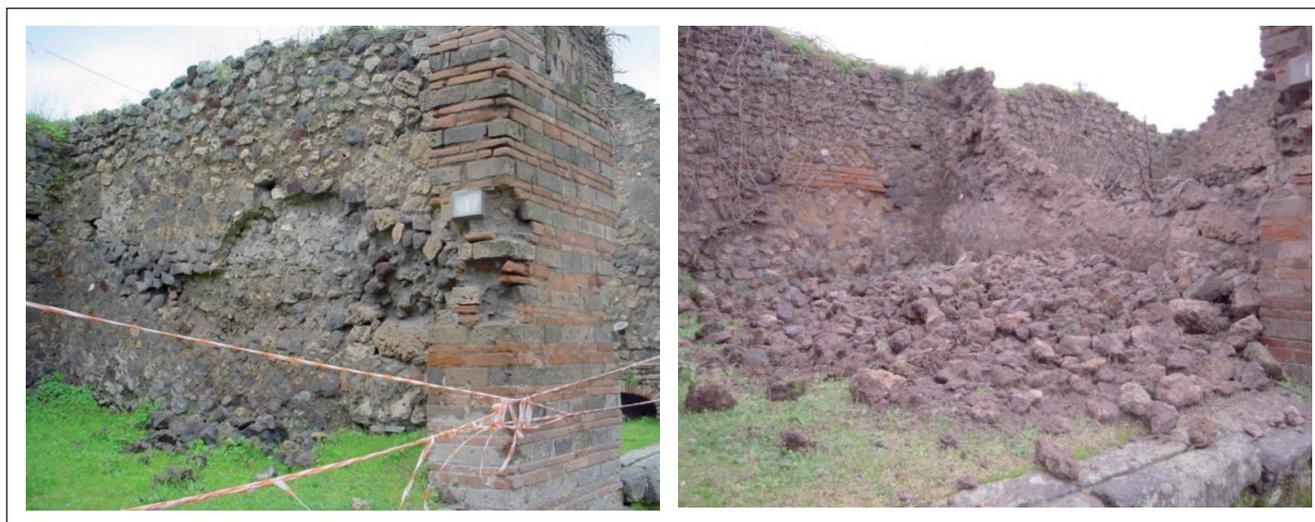
**FIGURE 1** Wall in Regio VII (Insula 2, No. 1), (a) before and (b) after the collapse
