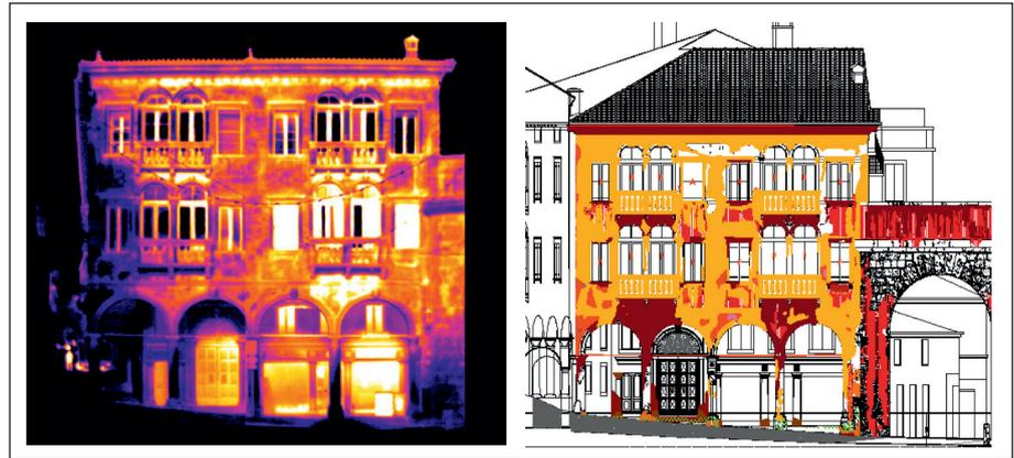
**FIGURE 8** Palazzo Todesco. Crack pattern survey of the external west side and distribution of the pulse sonic velocity at a column of the porch
