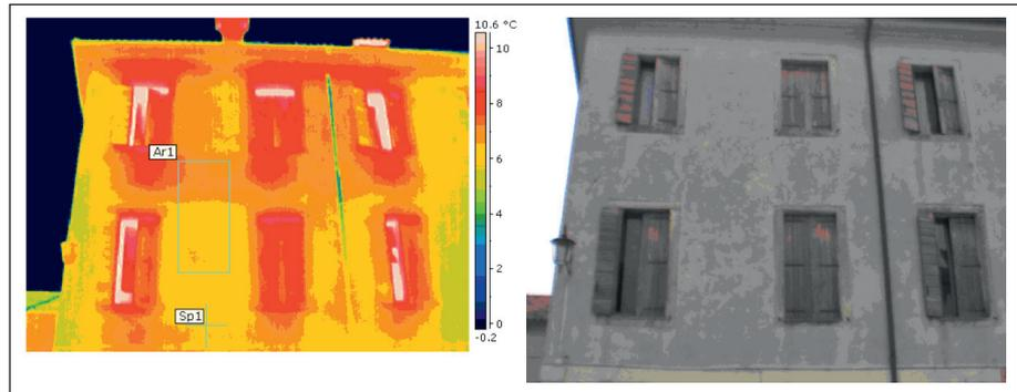
**FIGURE 13** Lower part of the façade in the morning. The earlier door place can be seen between the window and the door
