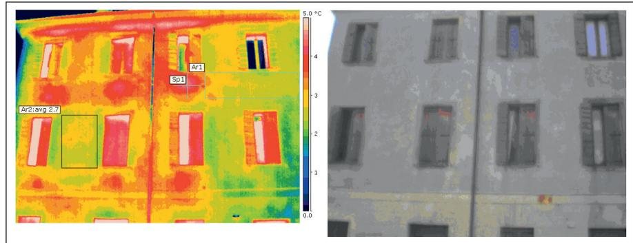
**FIGURE 12** The same façade during sun radiation. The external heat source removes the structural details
