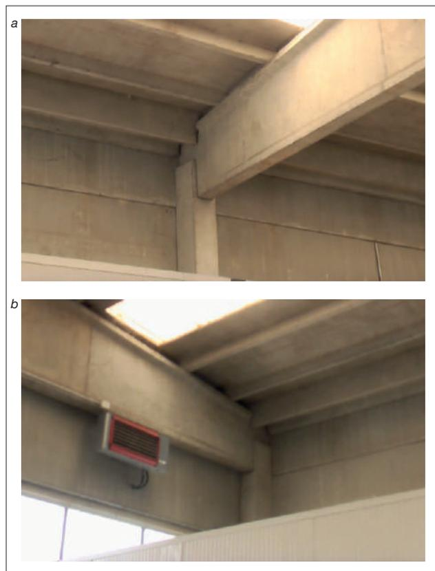
**FIGURE 9** Undamaged structure: a) covering structure to beam connection; b) corner configuration
