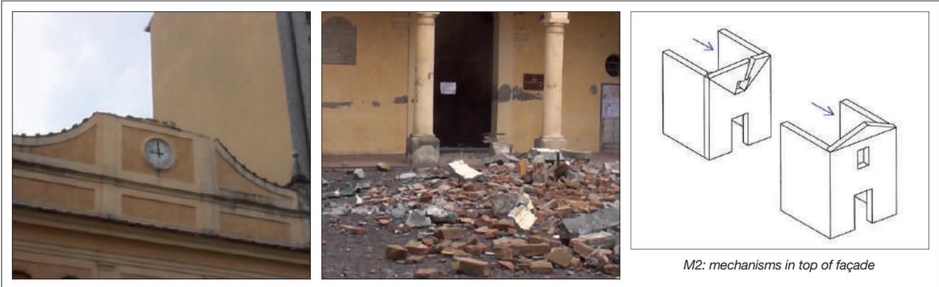
**FIGURE 11** Cento (Ferrara) historic centre: the Church of San Sebastiano and San Rocco (Convent of Friars Capuchins) and main collapse mechanisms
