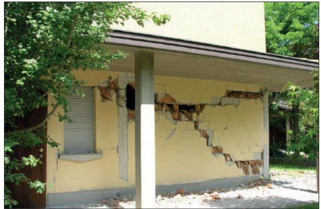
**FIGURE 17** Damage to ground floor wall
