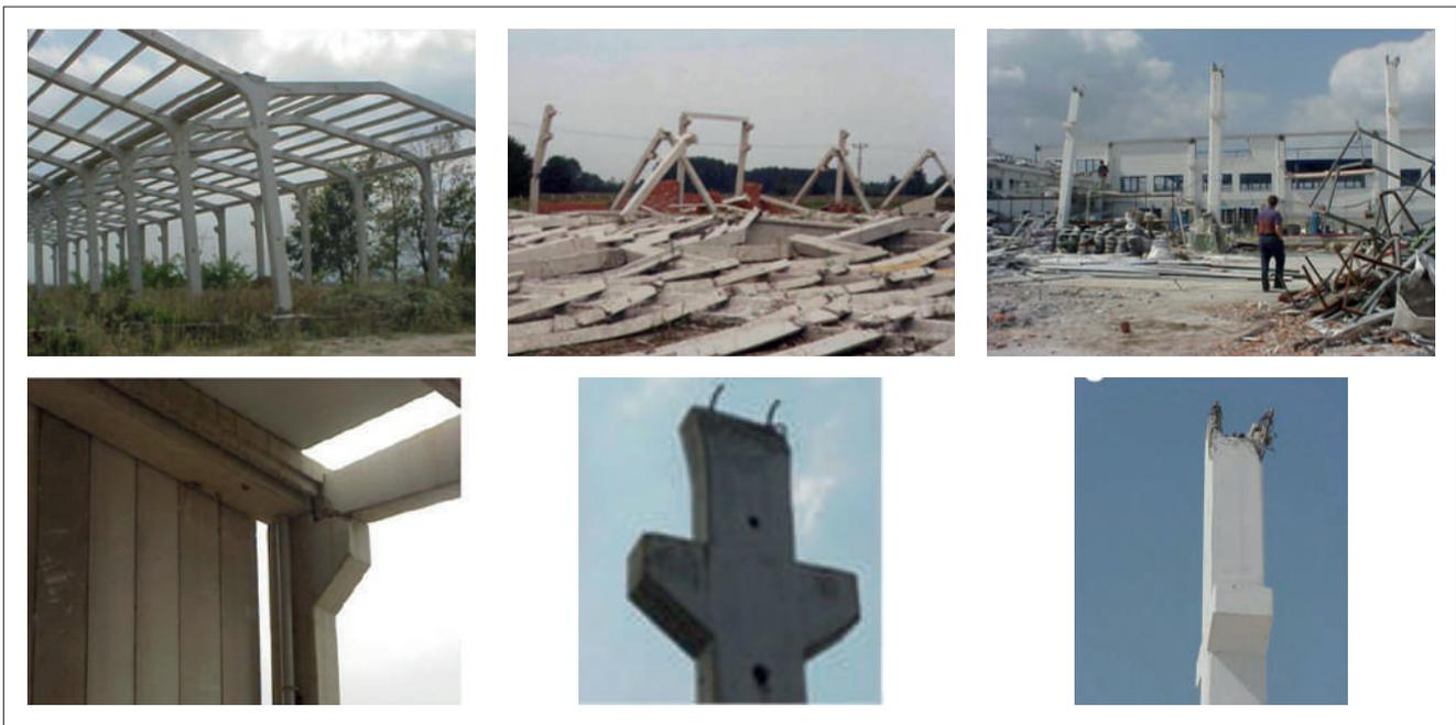
**FIGURE 17** P/p. r.c. structures, with different stages of construction and seismic behaviour, located in the epicenter area of the Kocaeli earthquake, and details of the connections [11-14]
