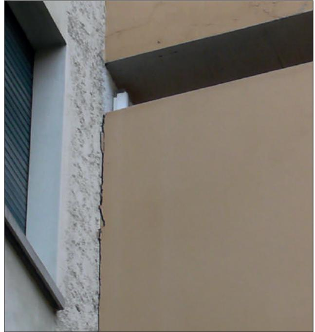
**FIGURE 27** Detachment of the parapet of some balconies
