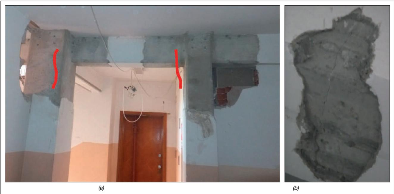
**FIGURE 32** Structural seismic damage: a) location of the cracks on the stair beams; b) crack detail
