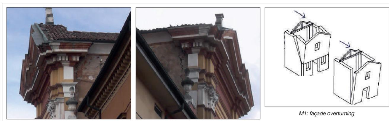
**FIGURE 10** Cento (Ferrara) historic centre: the church of San Filippo Neri and main collapse mechanisms
