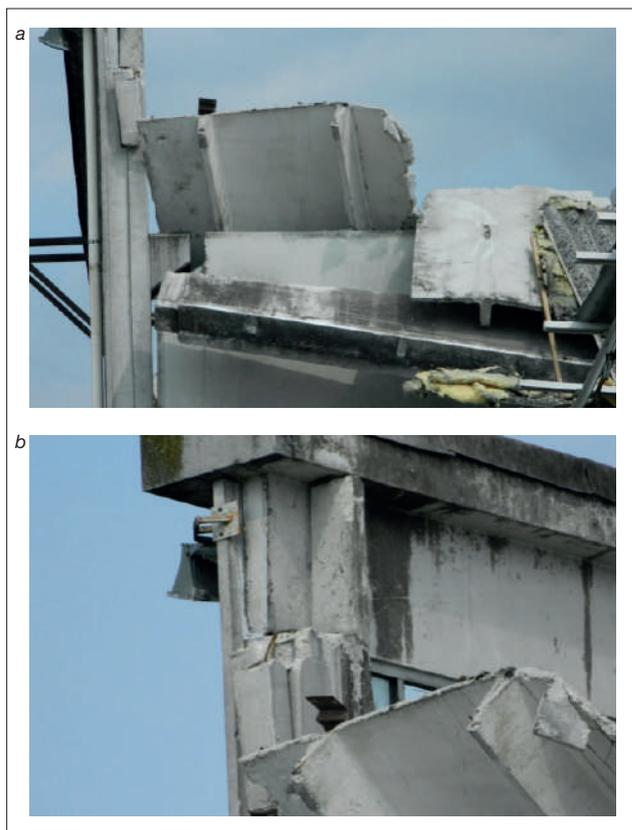
**FIGURE 10** Lateral toppling of the beam
