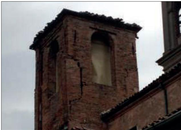
FIGURE 15 Separation and expulsion of the corner
