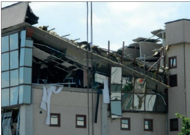
**FIGURE 7** Longitudinal slipping of the roof beams
