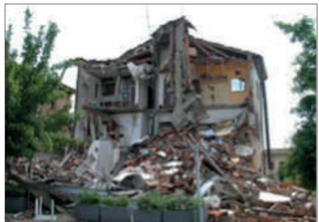
**FIGURE 4** The front part of the building has completely collapsed; the damage grade is 5
