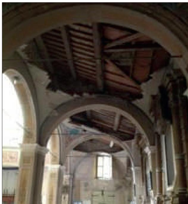
FIGURE 5 The collapsed vaults of the left nave
