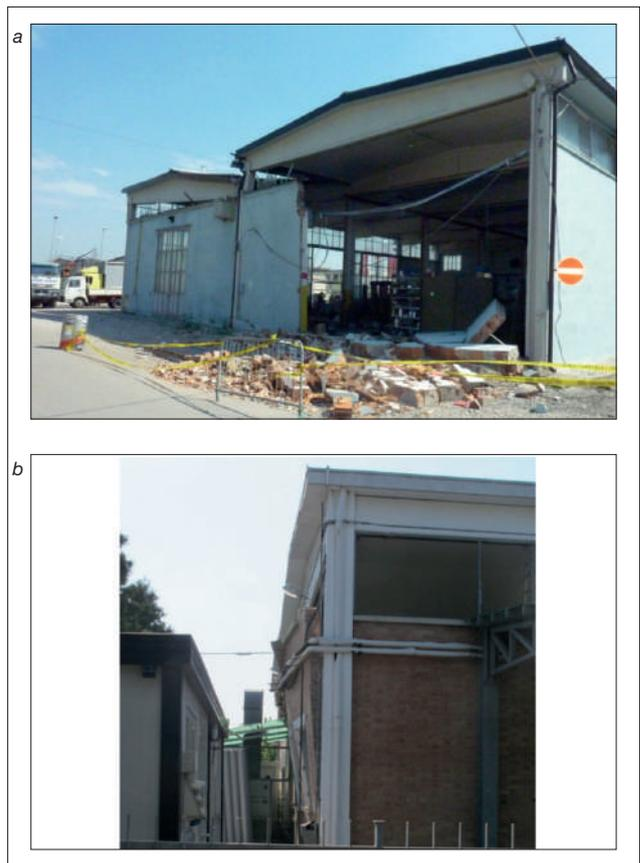
**FIGURE 14** Solid brick cladding damage
