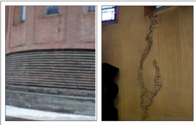
FIGURE 16 Subsidence phenomena: a) external view; b) internal view
