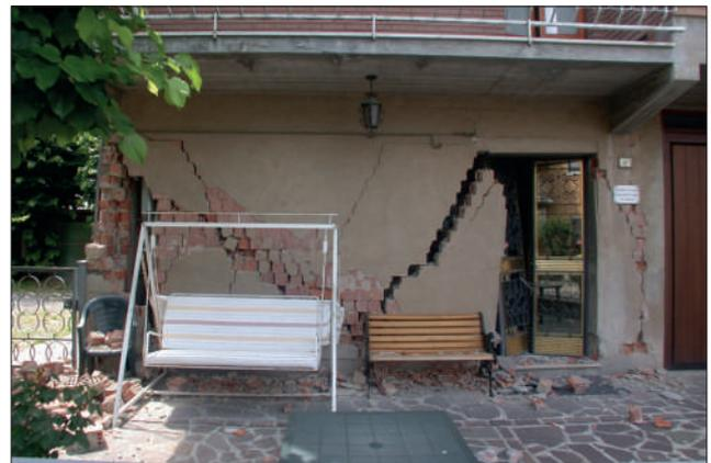
FIGURE 13 Serious failure of the walls, the damage is grade 4
