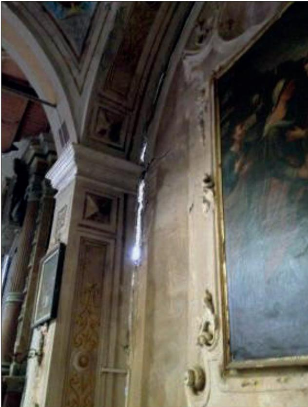
**FIGURE 13** Overturning mechanism of the walls on the left nave
