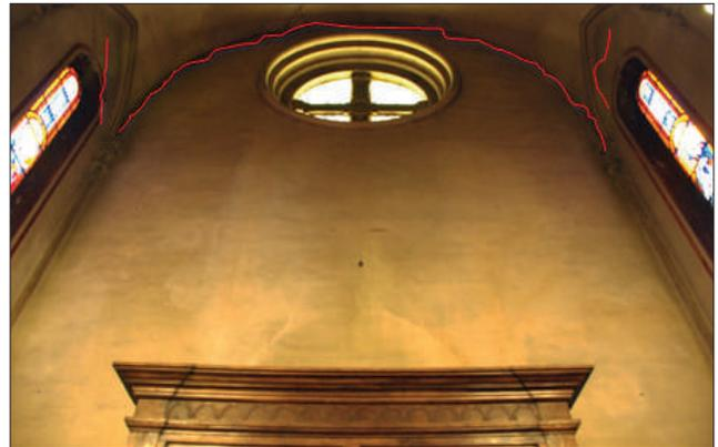
FIGURE 17 Façade overturning mechanism (M1), internal view
