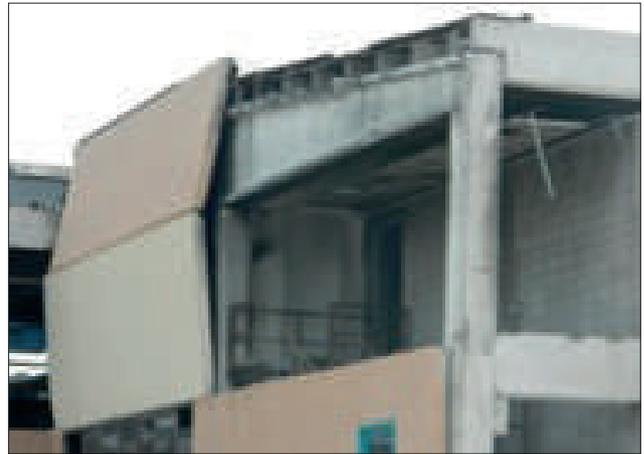
**FIGURE 13** Detachment of the external wall
