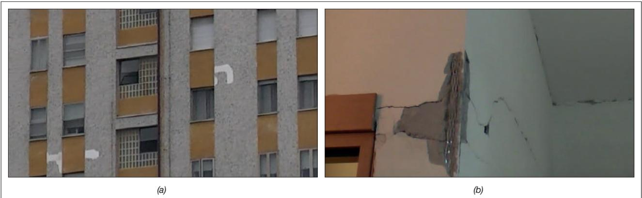
**FIGURE 33** Non-structural seismic damages: a) façade covering layers; b) partition walls
