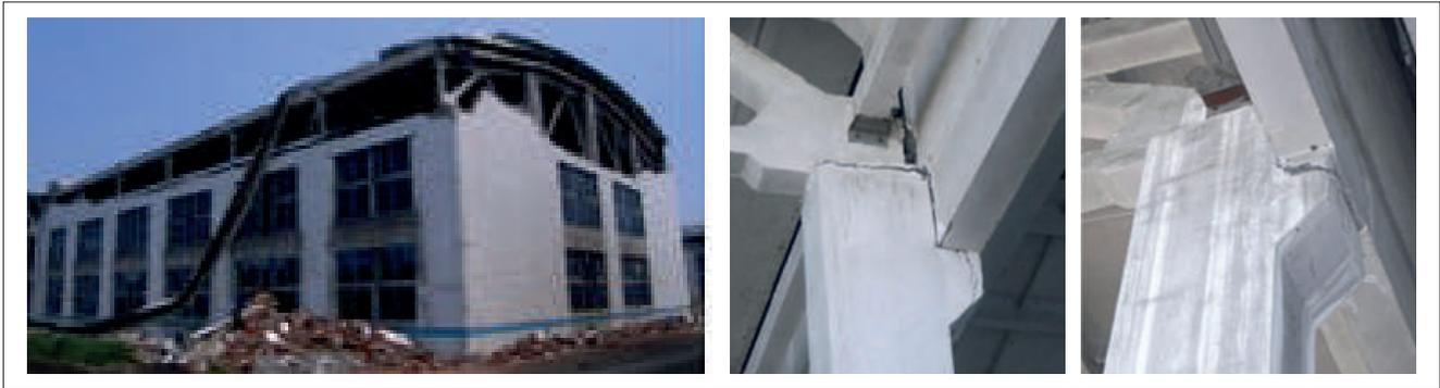
**FIGURE 18** Damage and partial collapse of the Xiting Package Ltd. Factory complex in Mianzhu City, Wenchuan, China [15]
