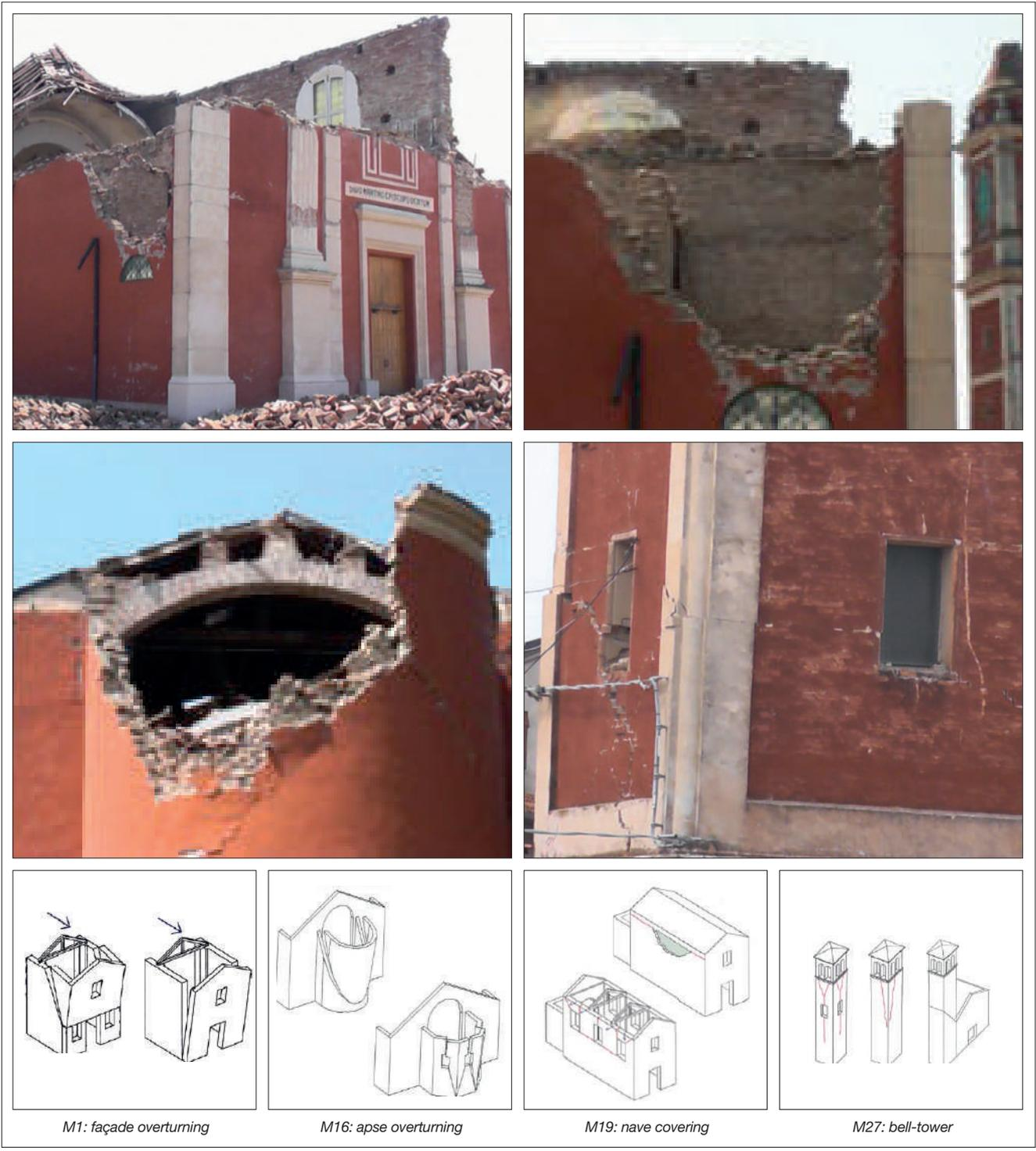
**FIGURE 5** Damage in the San Martino di Tours church and bell-tower in Buonacompra (Cento, Ferrara) and main collapse mechanisms
