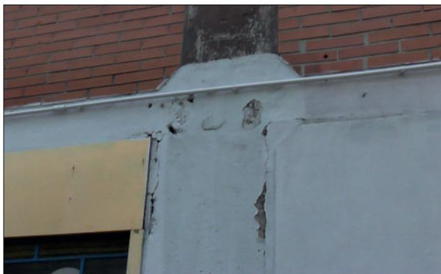
**FIGURE 28** Separation between cladding and structure elements
