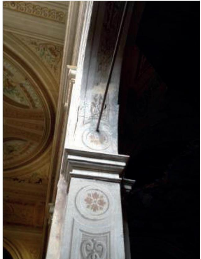
**FIGURE 14** Crack and translation on the arch
