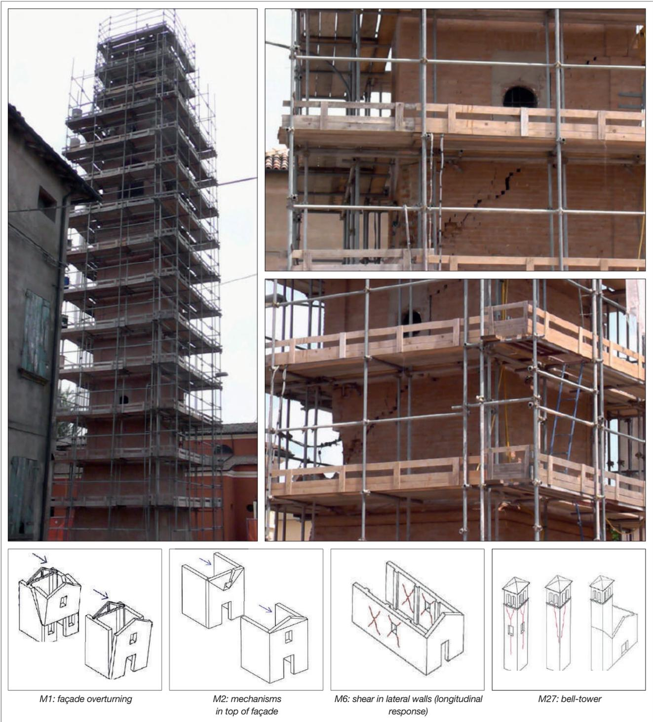
**FIGURE 8** Damage to the Sant'Anna church in Reno Centese (Cento, Ferrara) and main collapse mechanisms
