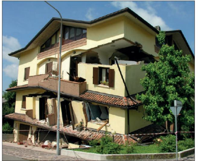
FIGURES 11-12 The soft storey has collapsed, the damage grade is 5
