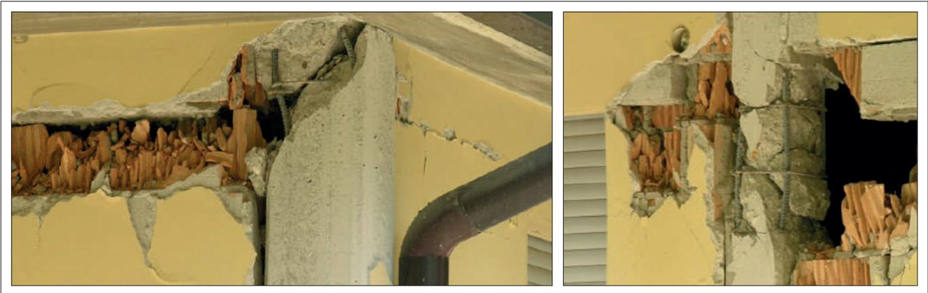
**FIGURES 18-19** Failure of RC columns
