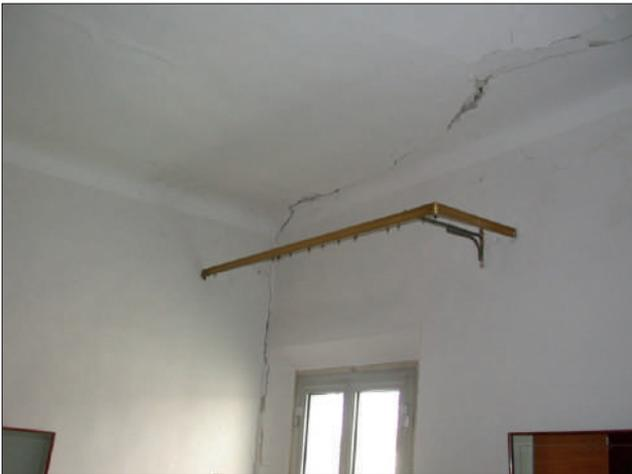
**FIGURE 10** Bondeno: damage of grade 2-3
