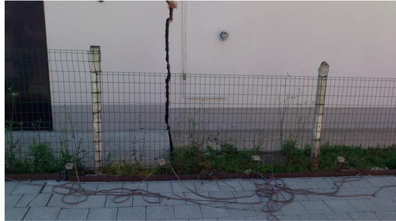
**FIGURE 3** Side view of the investigated building with structural damage. The residential building is situated in Via Argine Postale, 57, Mirabello village (Italy). Near the fence, the seismic cables with geophones can be seen
