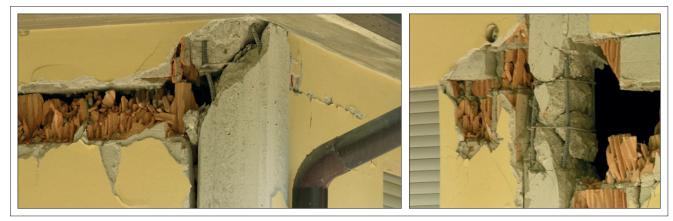
FIGURES 18-19 Failure of RC columns
