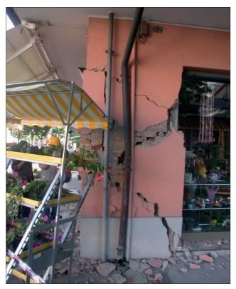
FIGURE 8 Heavy diagonal cracks with partial loss of connection between external walls (damage of grade 4)
