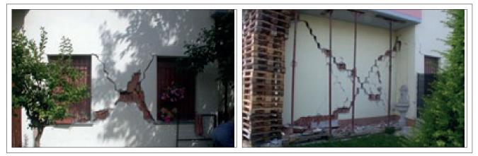
FIGURES 14-15 Large shear cracks on exterior walls; the damage level il 3
