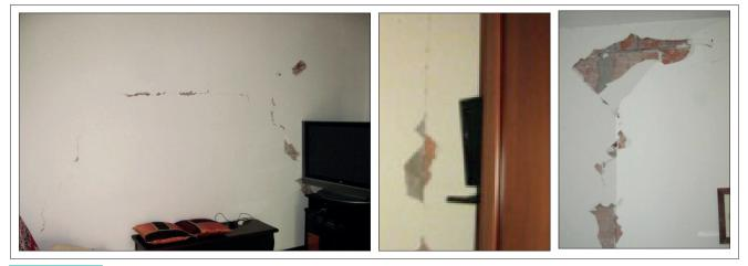
FIGURES 23-24-25 Damage to the partition walls
