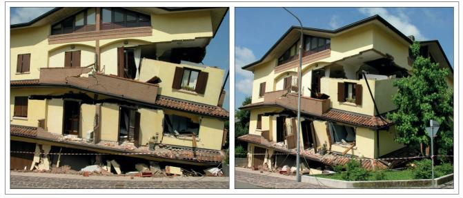
FIGURES 11-12 The soft storey has collapsed, the damage grade is 5
