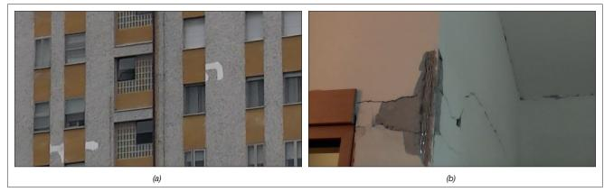
FIGURE 33 Non-structural seismic damages: a) façade covering layers; b) partition walls
