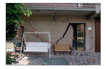
FIGURE 13 Serious failure of the walls, the damage is grade 4
