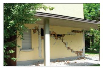
FIGURE 17 Damage to ground floor wall
