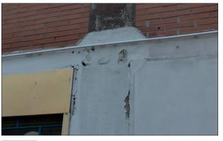
FIGURE 28 Separation between cladding and structure elements
