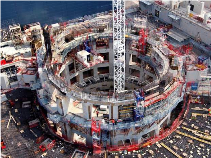
Fig. 3 Tokamak Building bio-shield under construction Source: courtesy of ENGAGE
