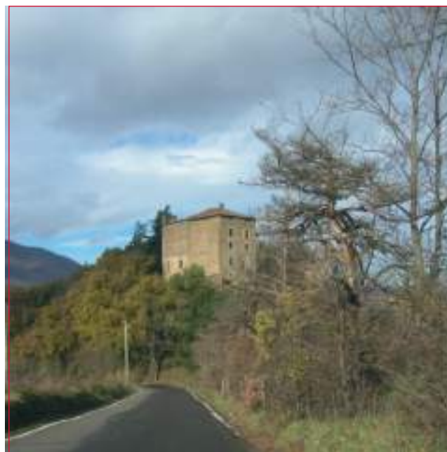
FIGURE 4 South view of the complex
