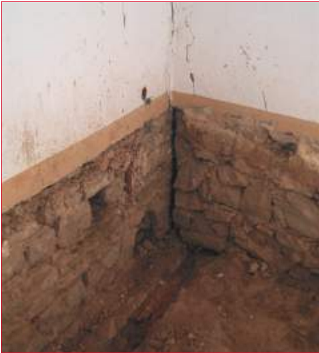
FIGURE 27 Remains of the ancient wooden tie
