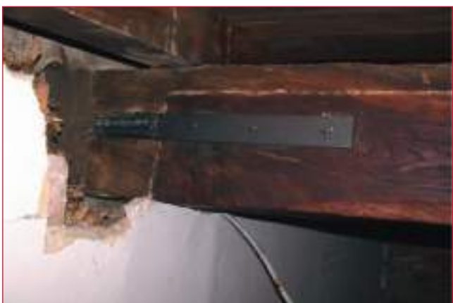
FIGURE 33 Connection floor-wall
