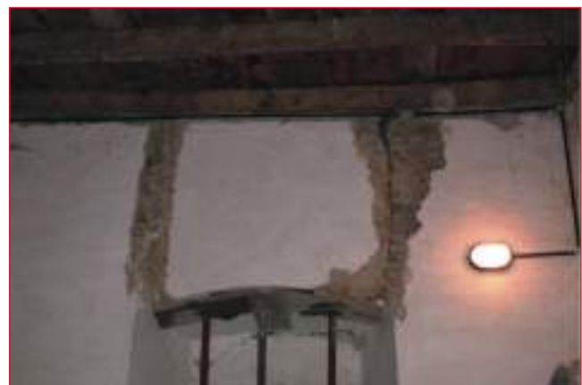
FIGURE 19 Detachment of walled-up window
