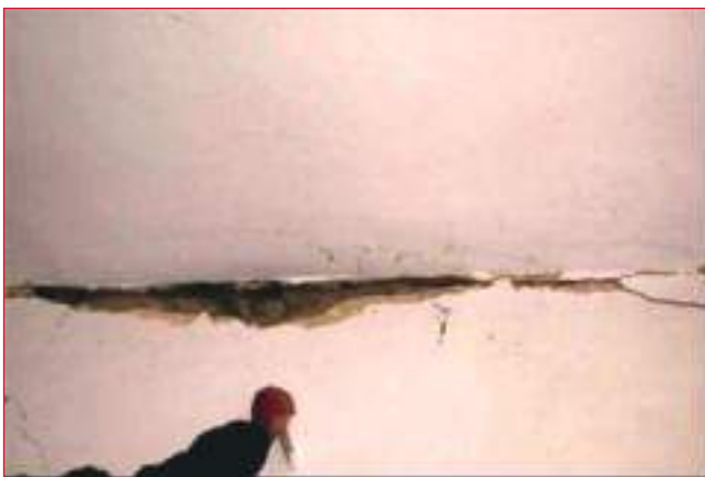
FIGURE 17 Wall-floor detachment
