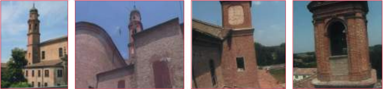
FIGURE 12 Church of San Giovanni in Municipality of Bondeno: view of the bell tower (ph. 1), helicopter in action for steeple image acquisitions (ph. 2), helicopter views (ph. 3&4)
