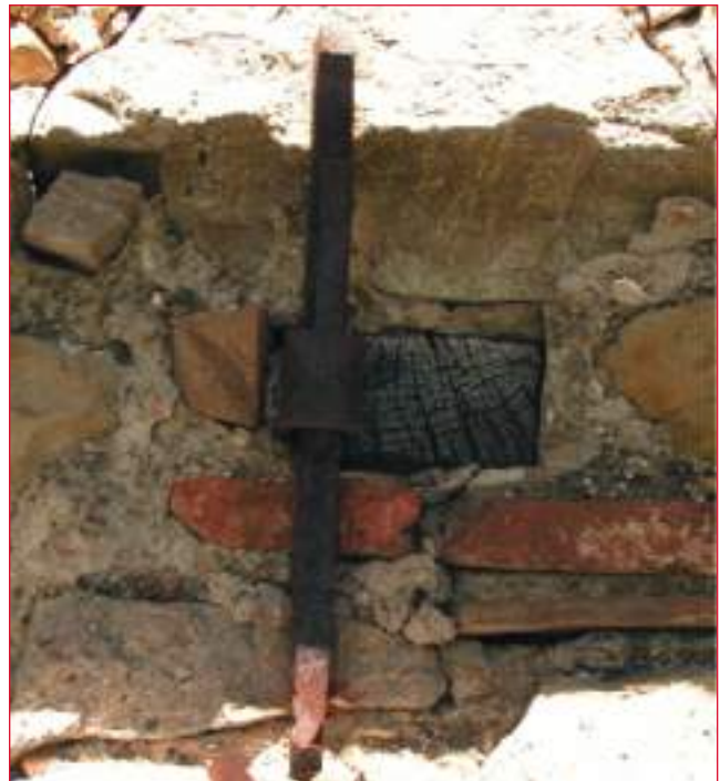
FIGURE 26 Wooden chain with metal anchor
