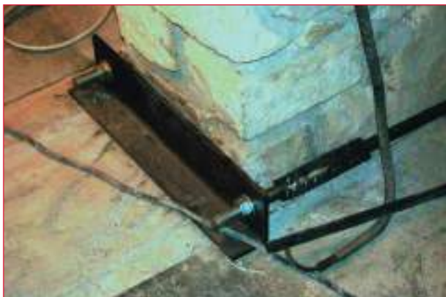
FIGURE 32 Example of internal tie-rod anchorage
