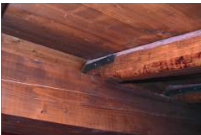
FIGURE 34 Metal connections to roof elements
