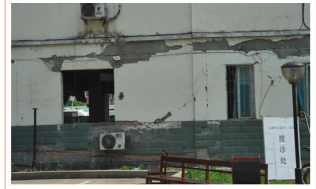
**FIGURE 11** The two buildings without seismic isolation in the Lu Shan County Hospital
