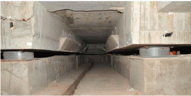
**FIGURE 19** Base isolation system in a retrofitted school
