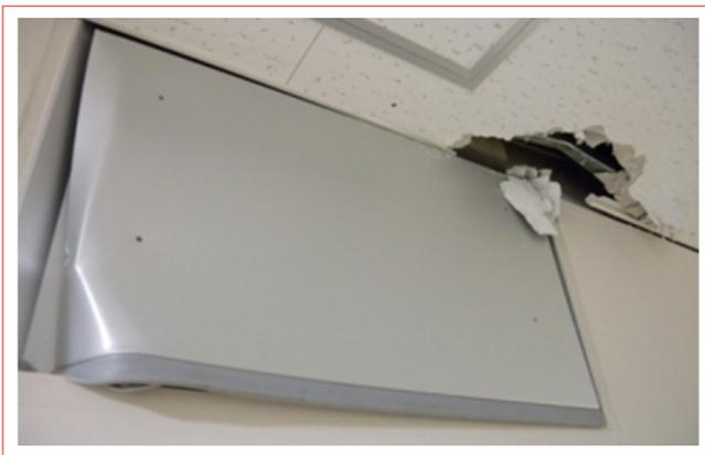
**PHOTO 3** Damage to cover panel
