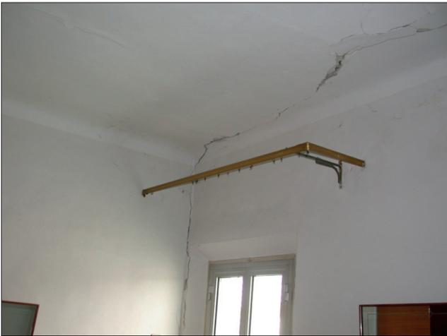
**FIGURE 10** Bondeno: damage of grade 2-3
