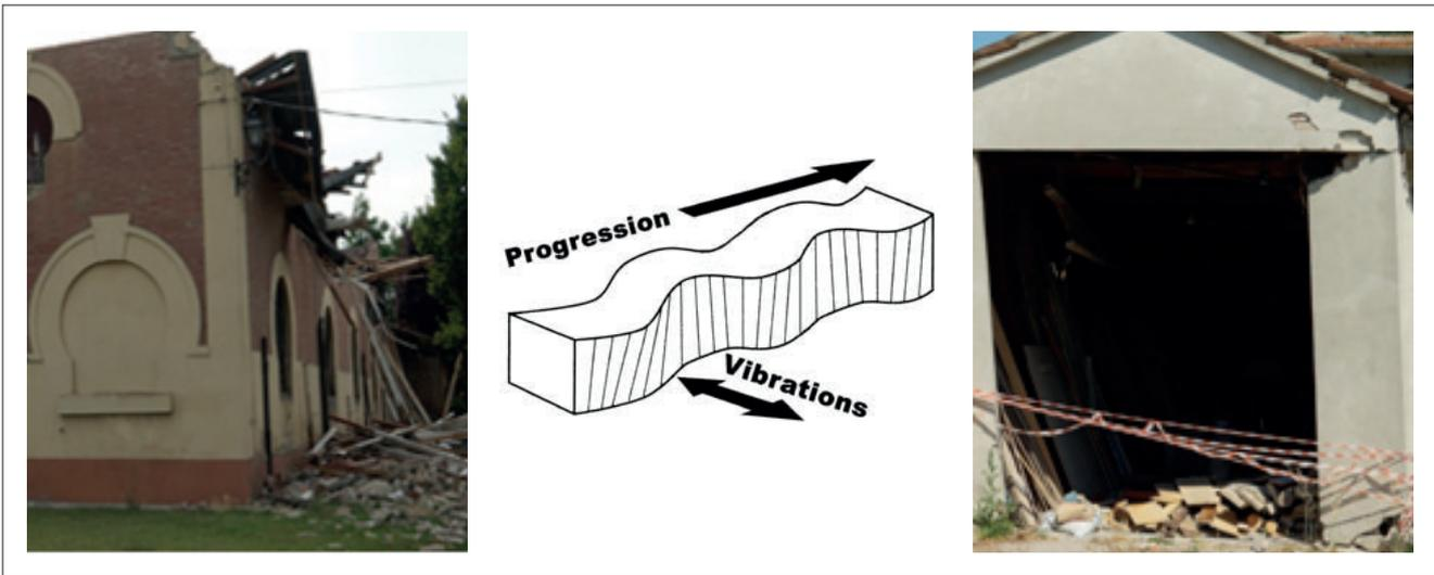
**FIGURE 14** Deformation by P waves due to L wave: rural buildings damaged in the Sant'Agostino area
